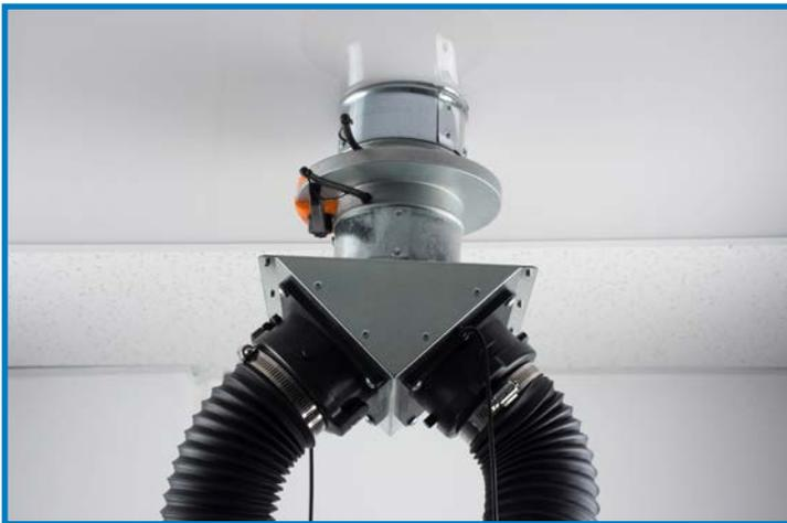
M49D100 iris damper connected to a V-box
